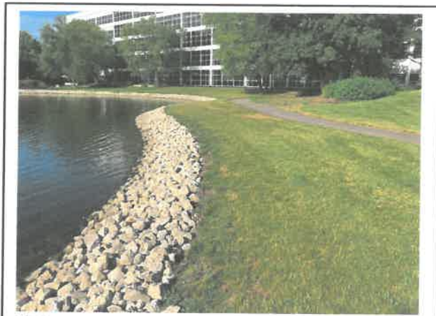
Photo 2: Stone toe stabilization.
