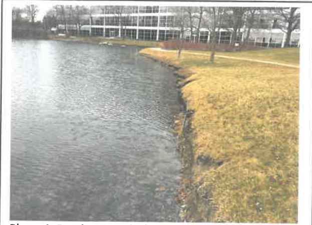
Photo 1: Pond erosion before stone toe stabilization.
