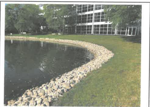
Photo 4: Stone toe stabilization.
