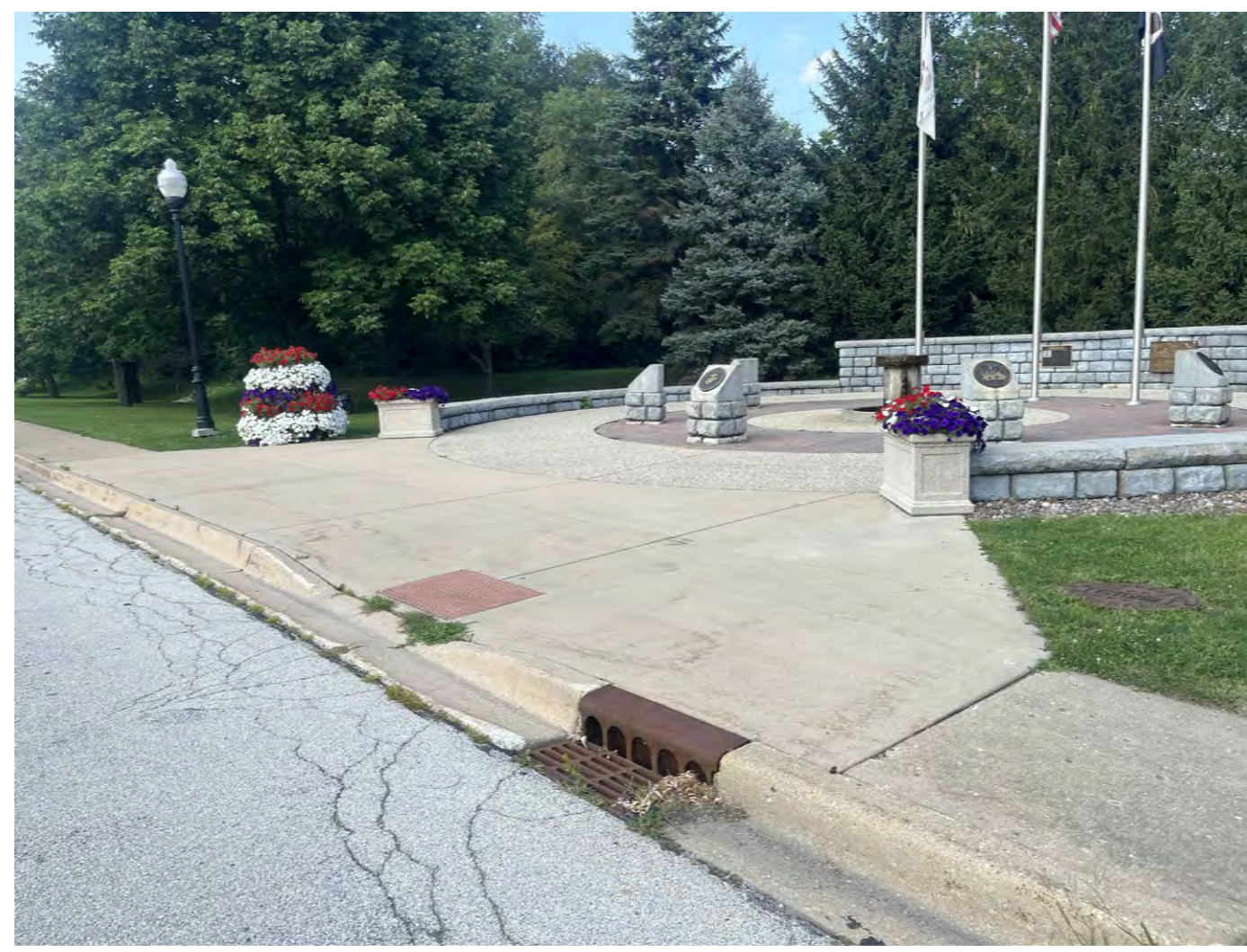
① EXISTING PLAZA OVERVIEW
