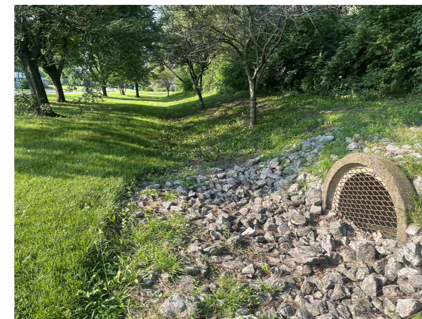
⑮ SWALE LINE AND DRAINAGE
