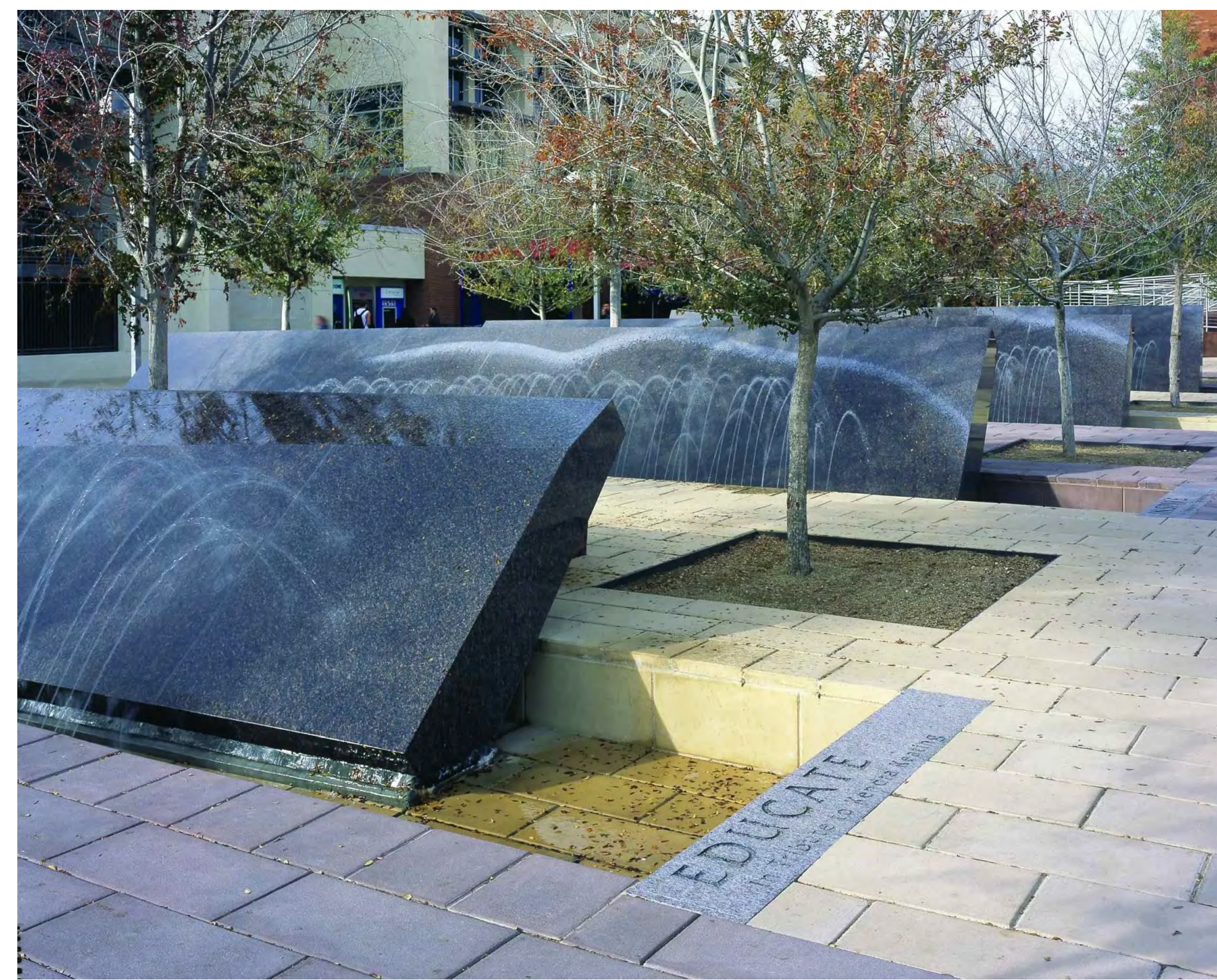
⑤ Engraved Granite Paver Around Fountain
