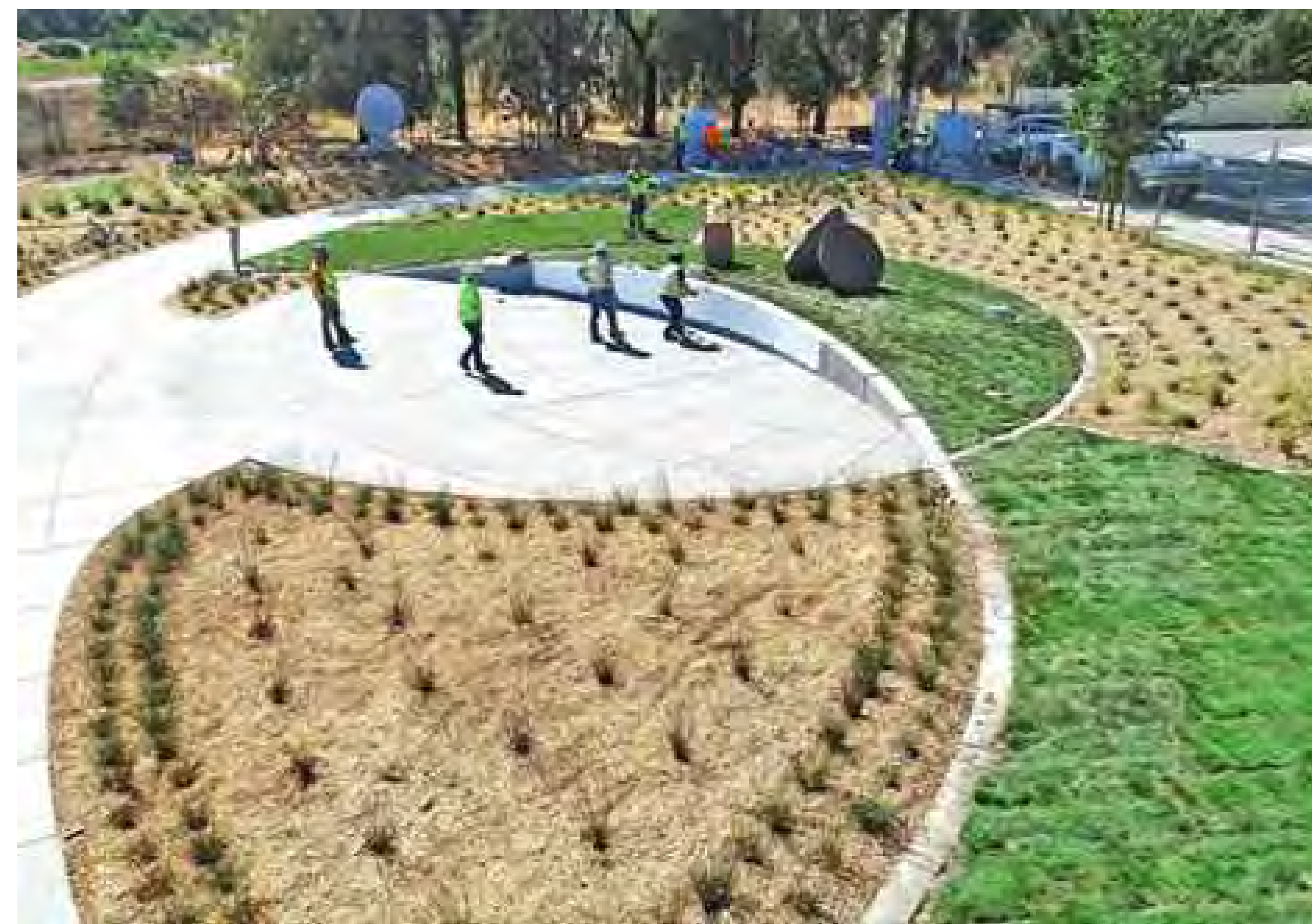
② Plantings and Curved Retaining Wall
