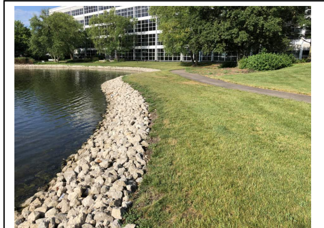
Photo 2: Stone toe stabilization.
