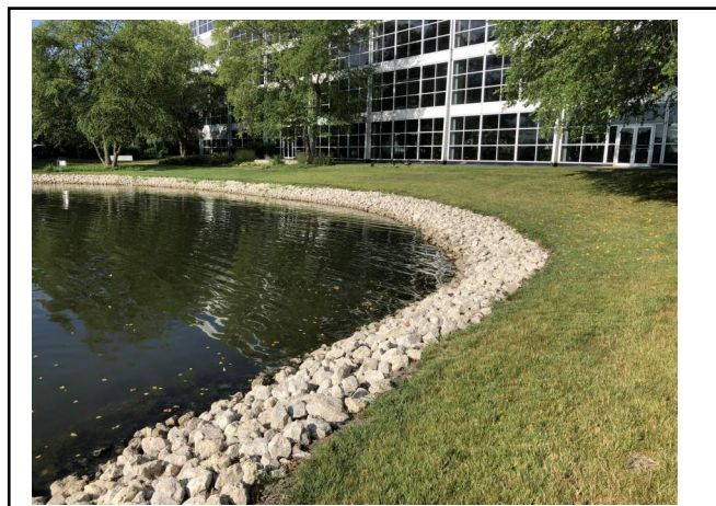
Photo 4: Stone toe stabilization.
