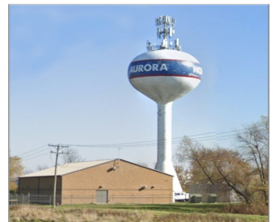
Central Water Tower
