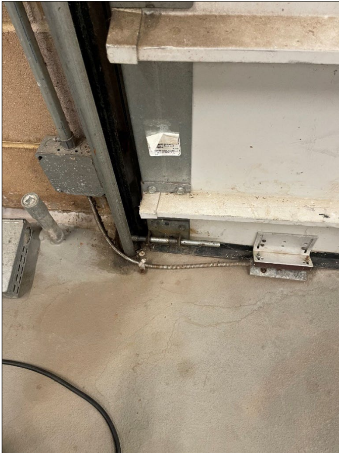
Overhead door floor contact
