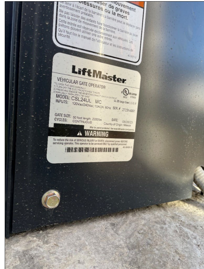
Gate Controller model – LiftMaster CSL24UL
