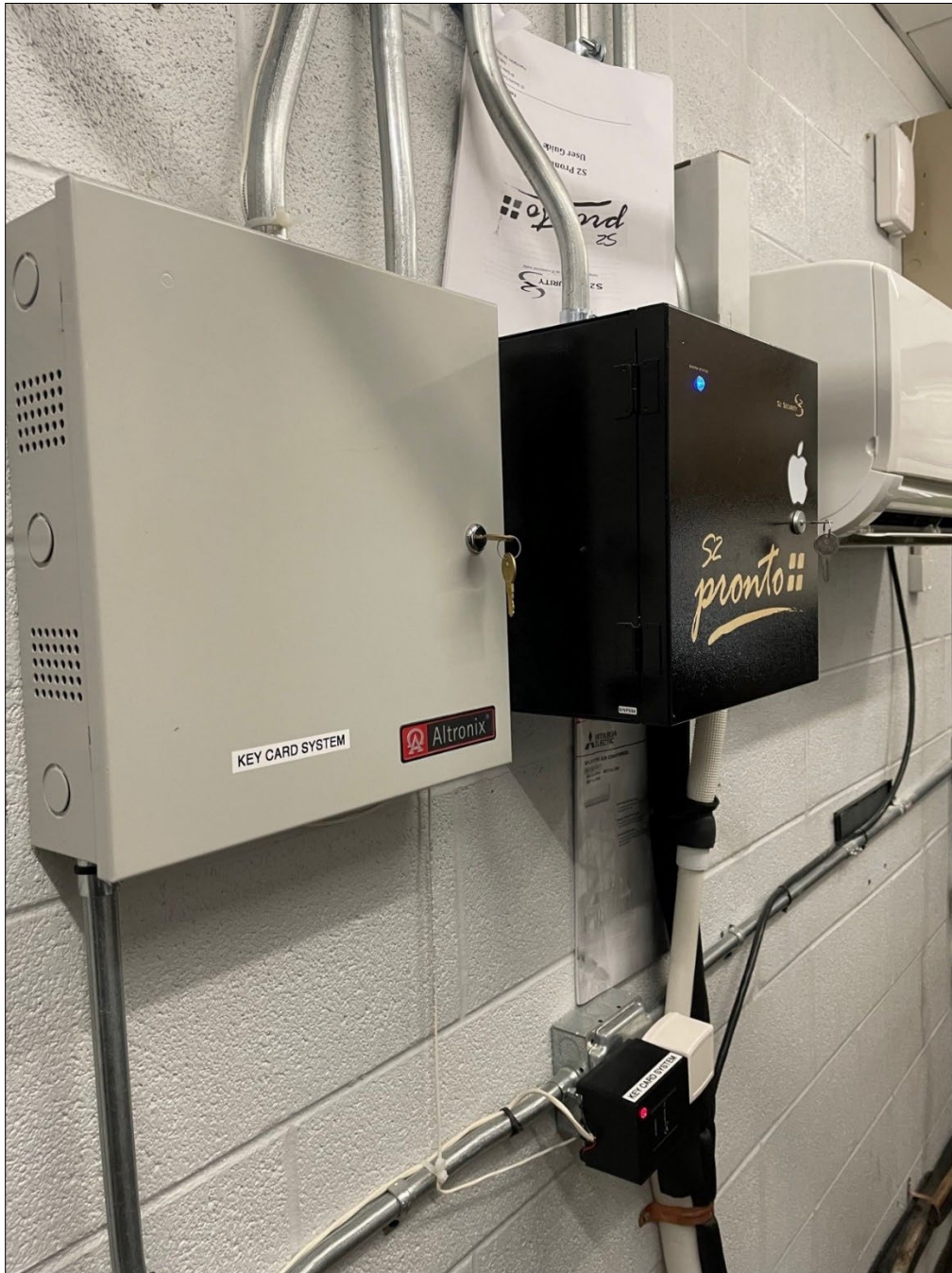
Current ACS Power Cabinet and S2 controller cabinet
