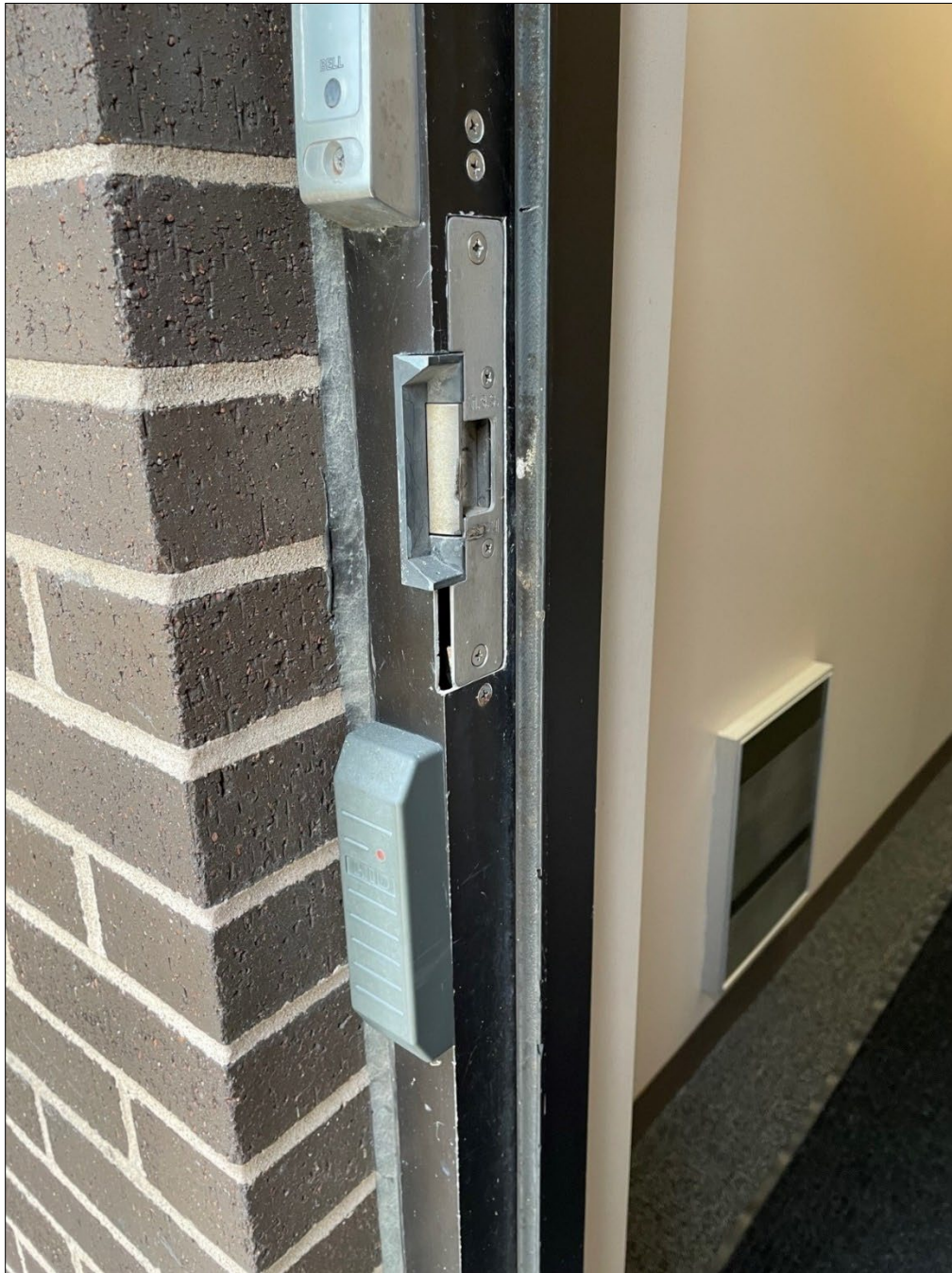
#3 Employee Entrance 1 - Current Door readers - Key pad is not being used.
