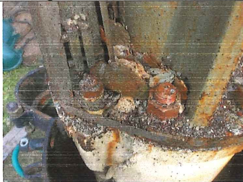
Shale fragments on bowl port body (just above motor)
