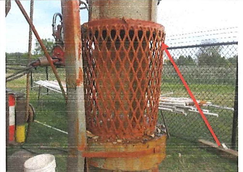
Suction screen clear except on fragment of shale
