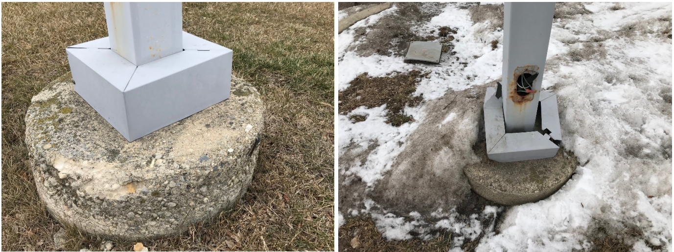
Hansen Blvd: spalled base, rusting pole, damaged bolt shield, missing handhole cover.
