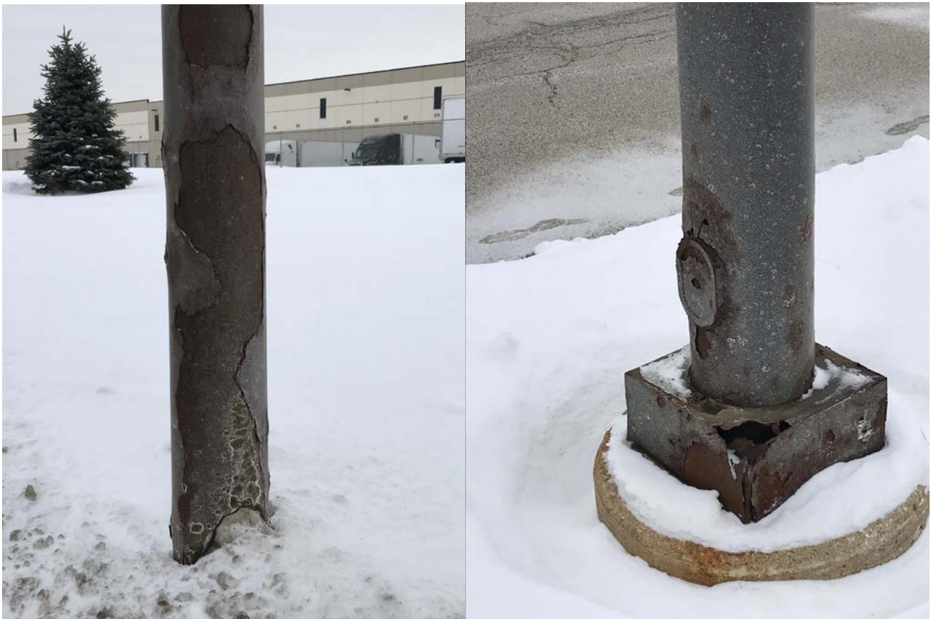
Orchard Gateway steel light poles: paint flaking from poles and rusted bolt covers.
