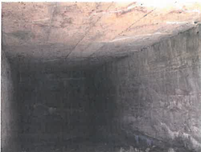
15. Typical cracking with efflorescence in substructure units and deck underside
