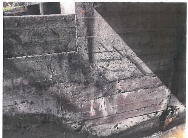
20. Showing deterioration of west spillway wall
