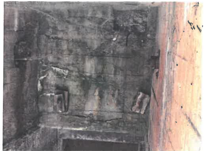
18. Discoloration and advanced deterioration of backwall at flow control structure
