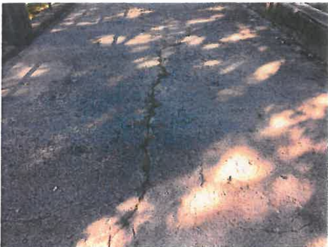
7. Typical map cracking and longitudinal crack in deck
