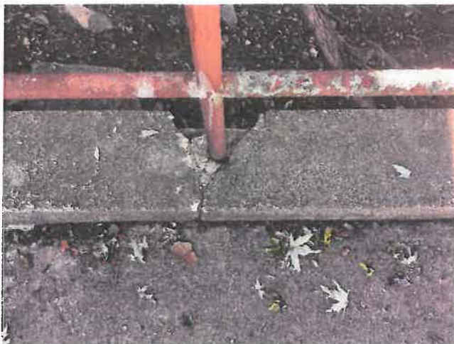
3. Spall in curb at railing post
