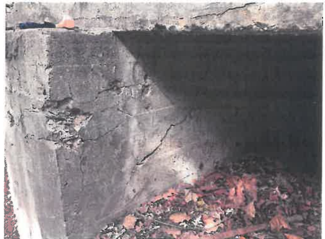
16. Typical cracks, spalls and delaminated concrete in piers
