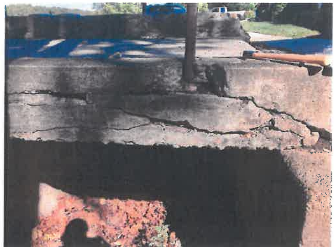
14. Significant deterioration of deck at southeast fascia
