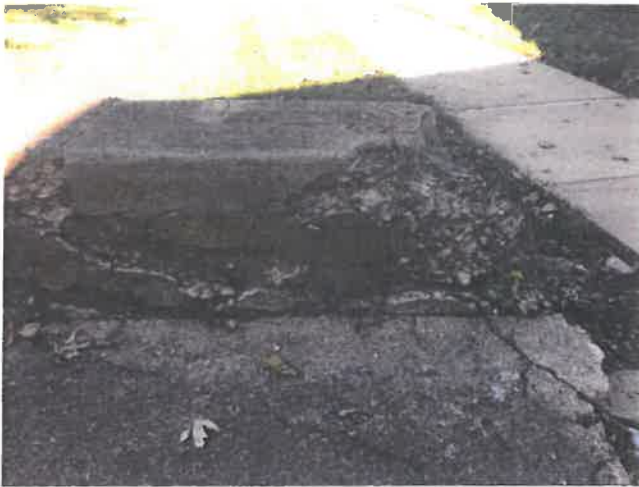
5. Typical deterioration of north curb
