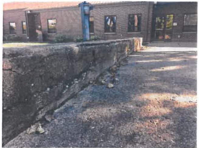
6. Typical deterioration of north curb
