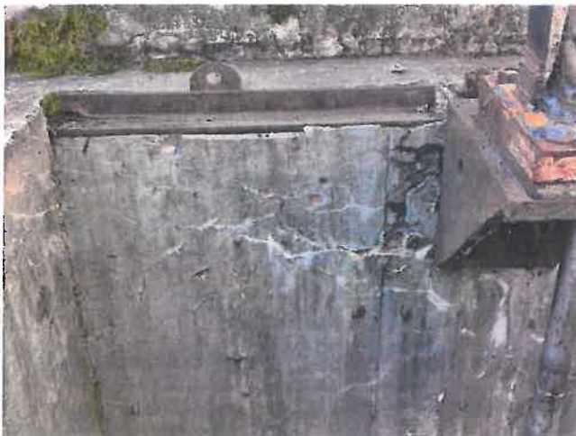
11. Deterioration of south wall at operating valve connection
