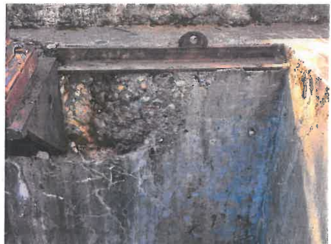
12. Deterioration of south wall at operating valve connection
