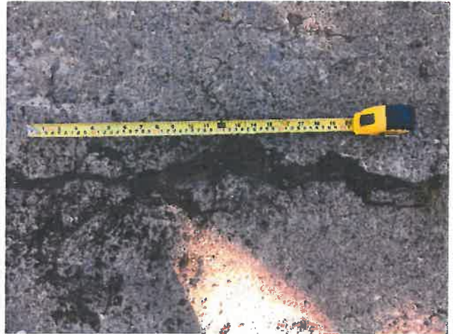
8. Deterioration of deck at longitudinal crack
