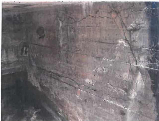
19. Showing deterioration of east spillway wall
