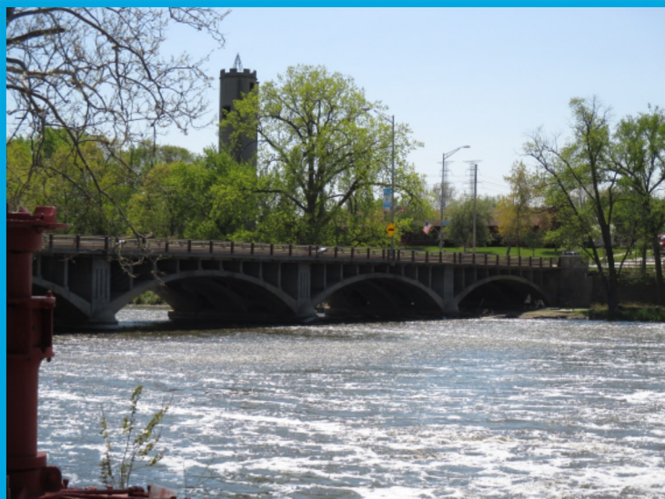
A view of State Street Bridge and the Fox River with the Silo rising in the background. The Village has plans to restore and light the silo in the future.
