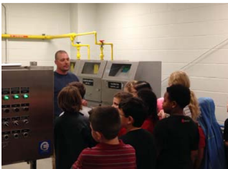
Mr. Barkei explaining to the students how the Village produces sodium hypochlorite (bleach) which is used as a disinfectant in the water treatment process.
